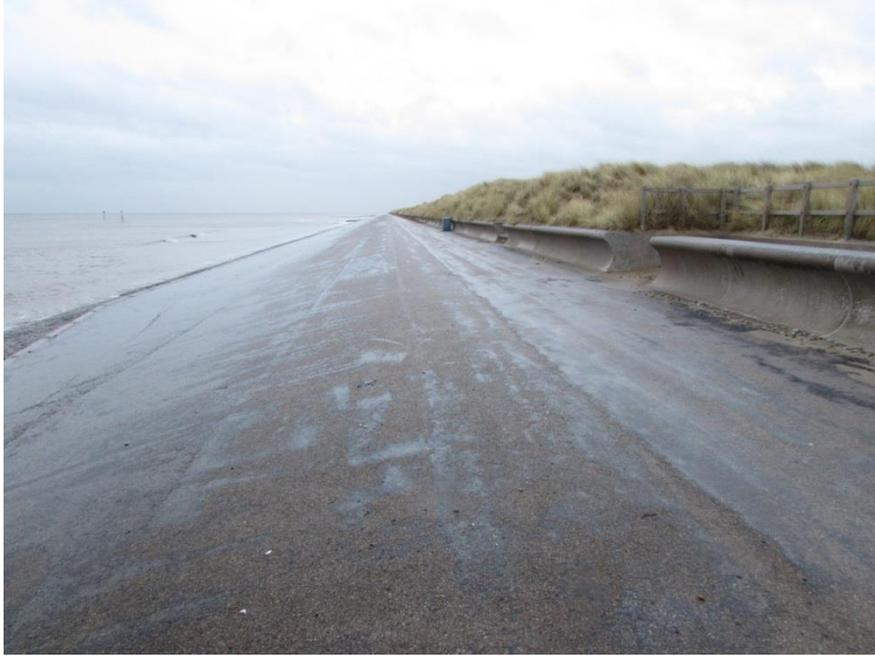
Figure 26. Gently sloping revetment and low wave return wall at Frith Beach, Prestatyn, which allows blown sand from the beach to reach the dunes
