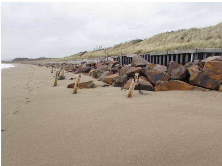
Figure 21. Rock armour and piling revetment at Abererch west, effectively cutting off the sediment transport connection between the beach and the dunes
