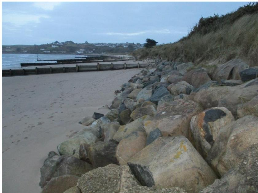
Figure 25. Rock armour and groynes used to protect the dune frontage at the southern end of Morfa Gors, Abersoch
